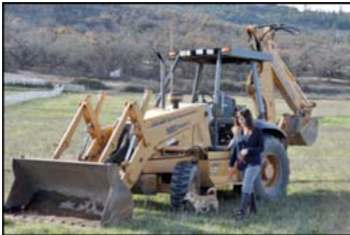
Accounting Manager Meagan Steahly touring around the construction site with demo dog Keen.
