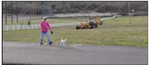
Volunteer dog walker Donna, passing in front of the new construction site, where Dogs for the Deaf's 18, 000 sq ft second training facility will reside.
